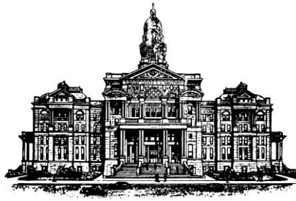
Tarrant County 1895 Courthouse
