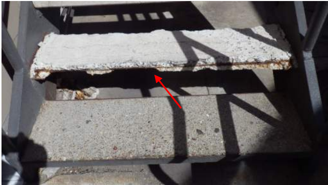
1968 deteriorated steps
