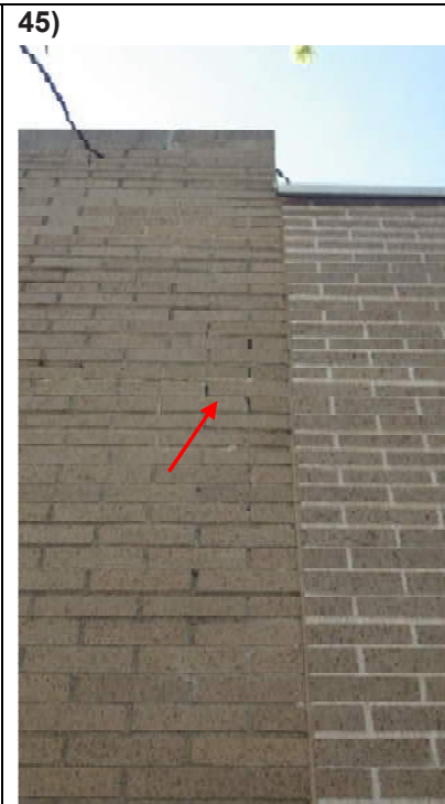
1972 precast wall at ramp
