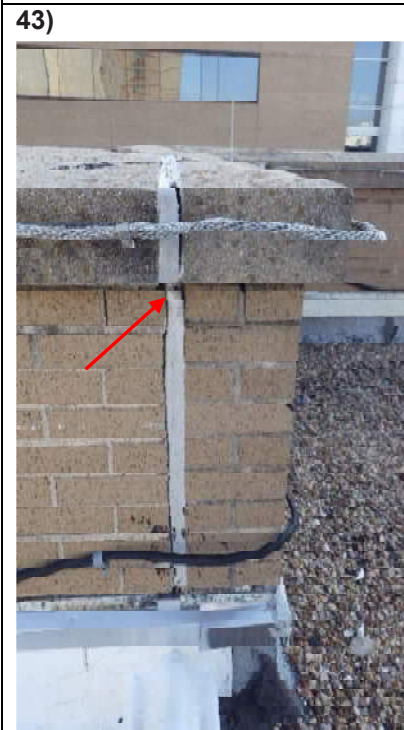
1972 parapet joint
