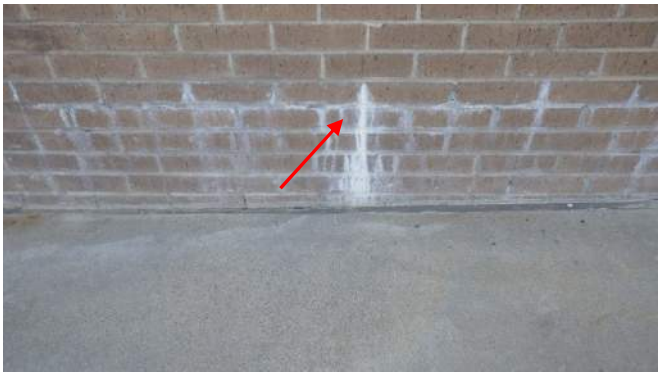
Plant weep holes at base of wall
