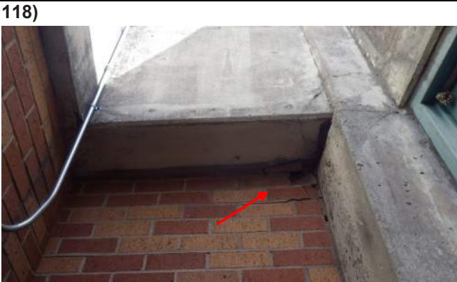
Old St Joseph Parking Structure
