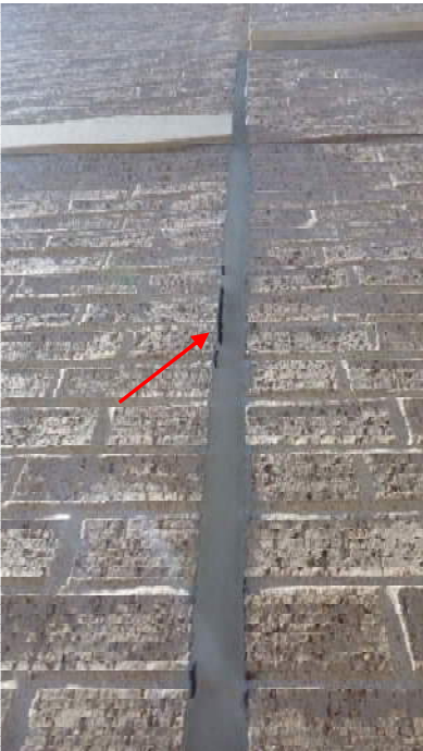
Pavilion Parking Structure joint
