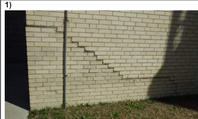
1939 north wing - cracking
