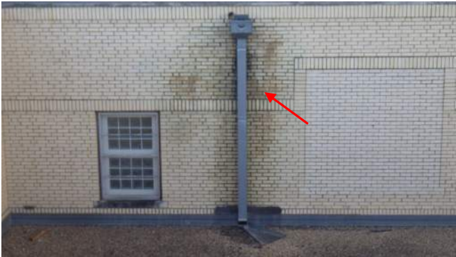
1939 moisture deterioration
