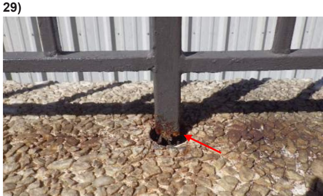
1968 deteriorating rail
