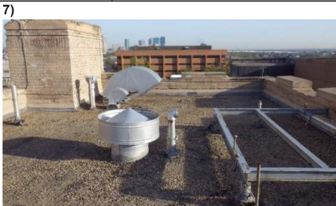
1939 penthouse roof - worn
