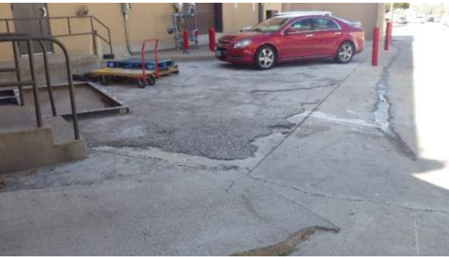
Receiving parking lot
