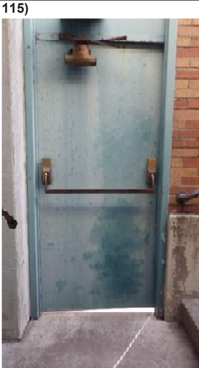
Old St Joseph Parking Structure
