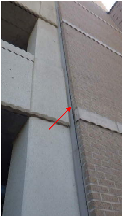
Pavilion Parking Structure joint
