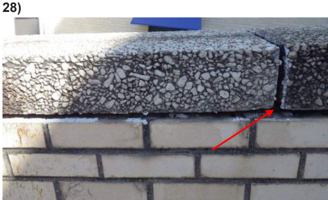
1968 precast wall at ramp – missing sealant
