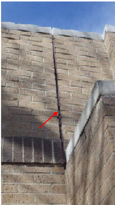
Tunnel joint sealant
