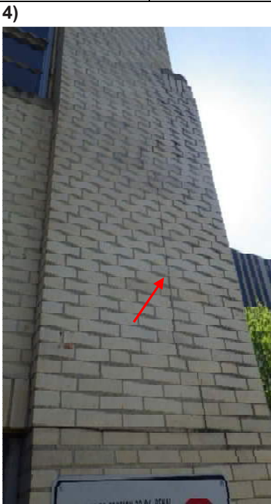
1939 north wing - cracking
