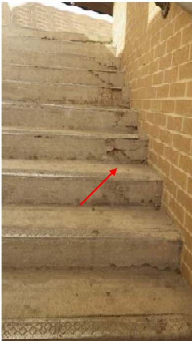
Entry Building exterior stairs
