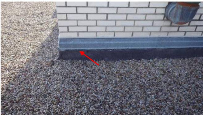
1959 / 1968 deteriorating flashing
