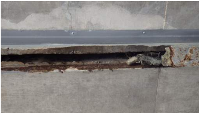
Old St Joseph Parking Structure
