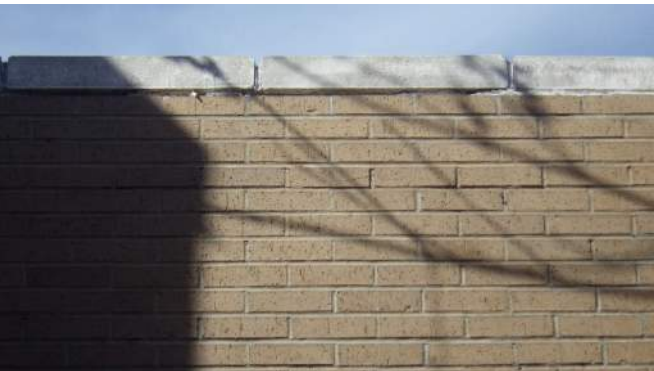
Tunnel parapet coping joint sealant
