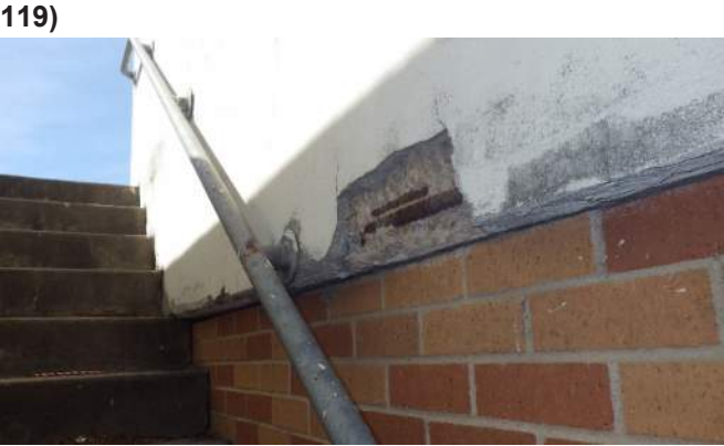
Old St Joseph Parking Structure
