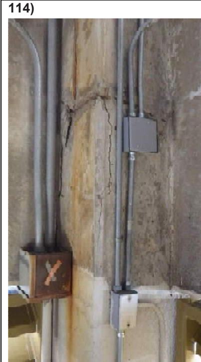
St Louis Street Parking Structure
