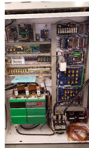
4. Typical Low-Supported, Problematic EC V800 Controls installed in 1995/96 on Units #8, 9, 12, 13, 14, 15, 19, 20, 21, 22 & 23. This Unit (#19) contains Obsolete Mentor II Drive
