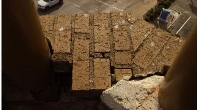
St Louis Street Parking Structure
