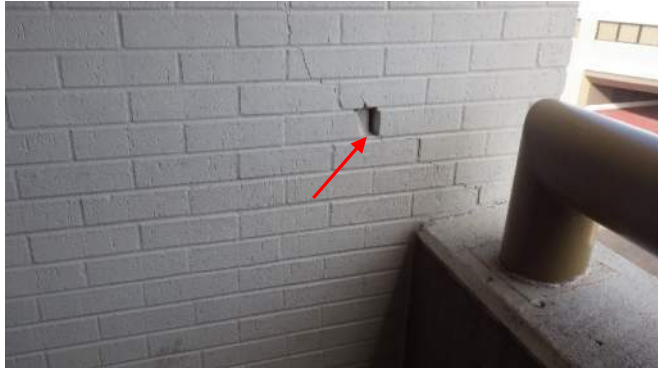
St Louis Street Parking Structure
