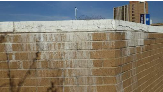
Trinity Springs screen wall
