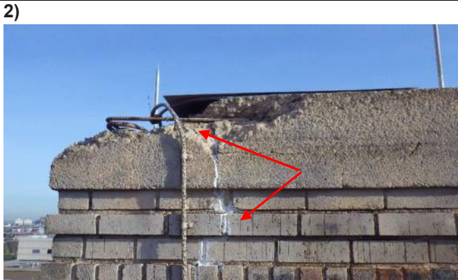
1939 penthouse cap - deterioration
