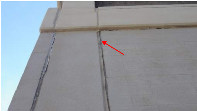
Pavilion Parking Structure joint
