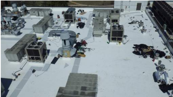
Pavilion roof replacement
