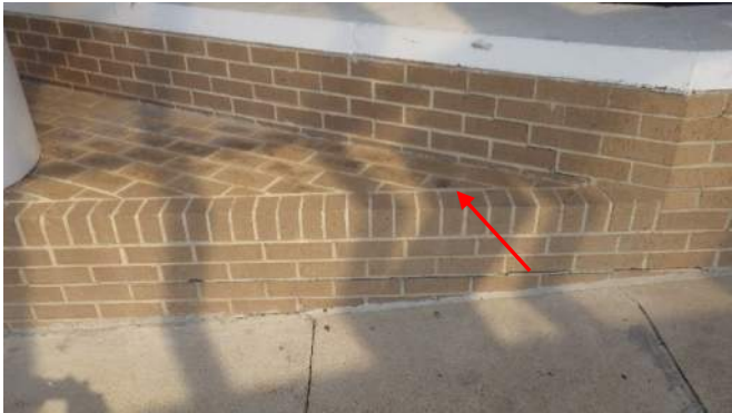
Entry Building retaining wall
