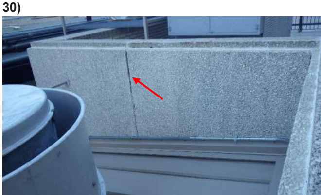
1968 precast wall – missing sealant
