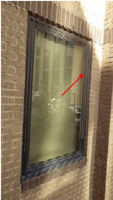
Tower Addition window sealant
