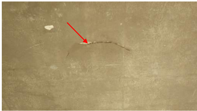
Old St Joseph Parking Structure
