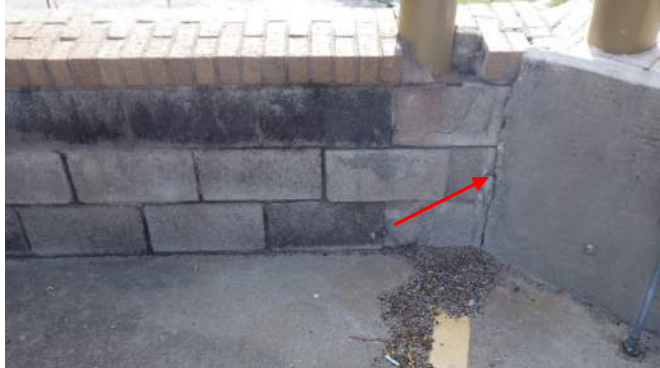
St Louis Street Parking Structure
