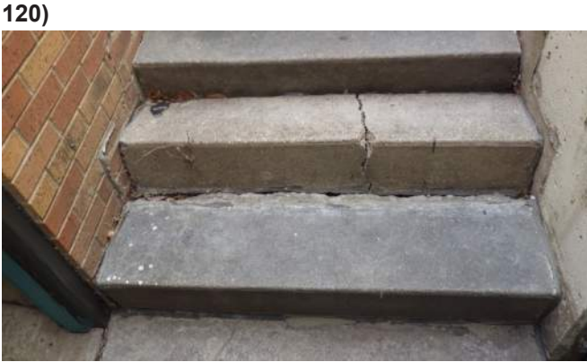
Old St Joseph Parking Structure
