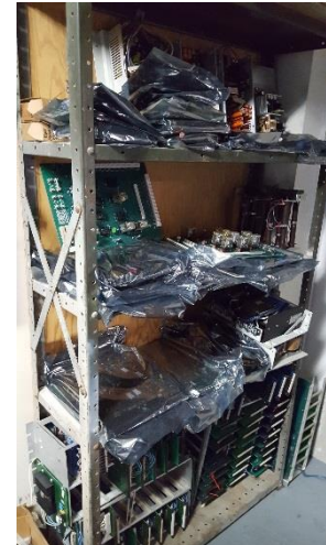
2. Stacks of Used Obsolete Boards to support Montgomery Ultron Units
