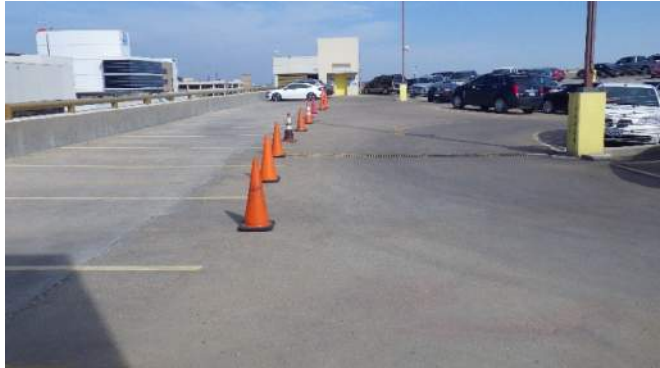
St Louis Street Parking Structure
