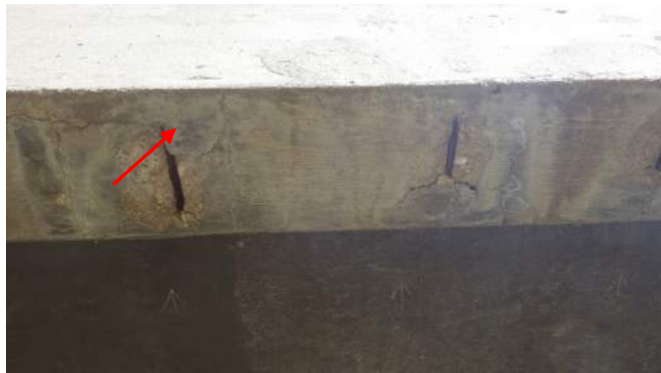
Old St Joseph Parking Structure
