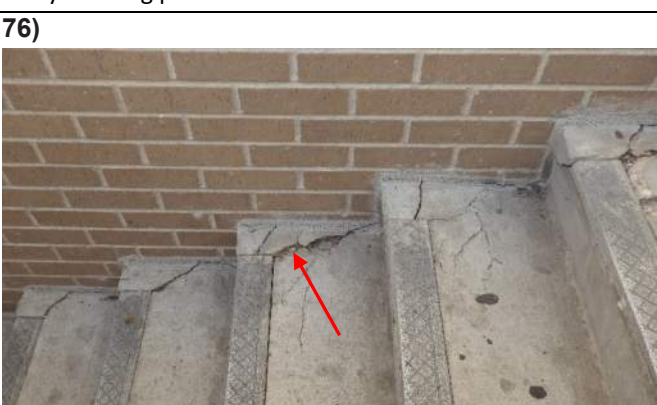
Entry Building exterior stairs
