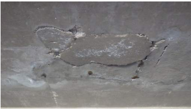
Old St Joseph Parking Structure
