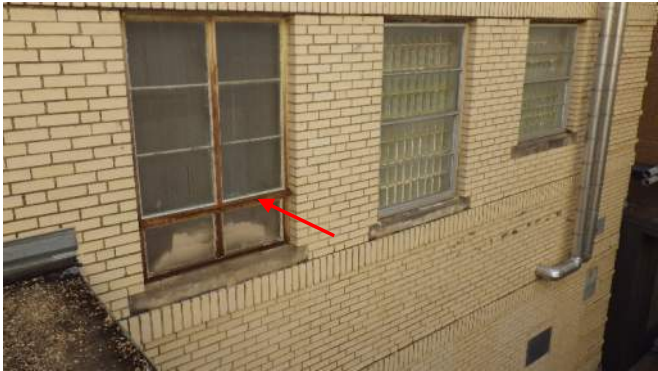
1939 window deterioration
