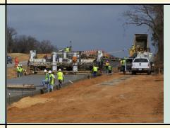
The FM 1938 contractor has laid first sections of concrete paving from Dove road to SH 114 and installed the pedestrian underpass within the last couple of weeks.
