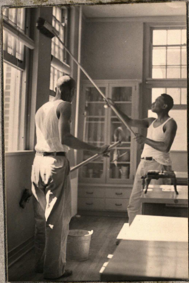
Custodians at Quinn School on a "Cleaning-Up Job"
