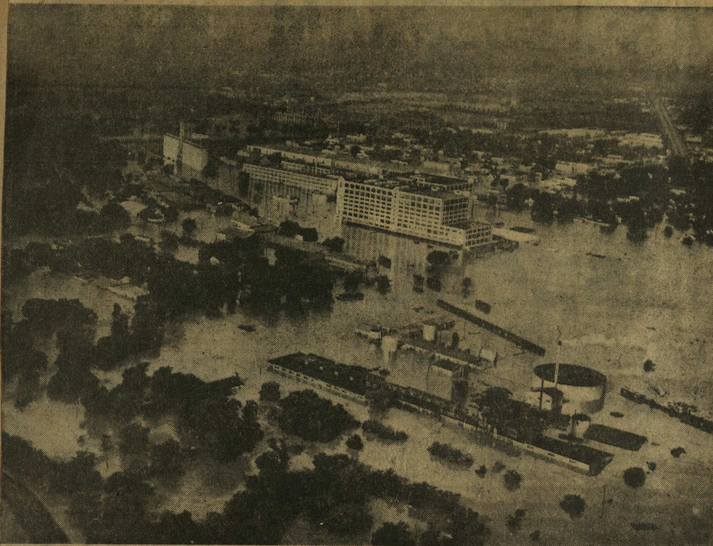
READY FOR REHABILITATION —Here's a typical job that confronted Fort Worth's citizens and municipal government, busy Wednesday with rehabilitation after
