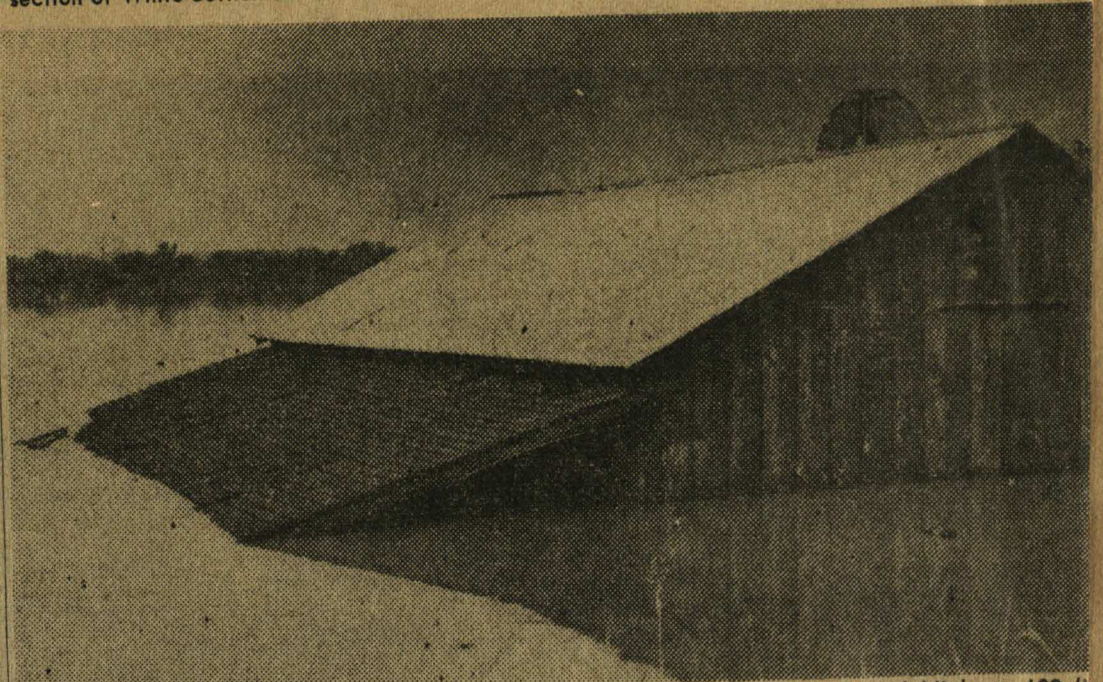
DIVERS would have been needed to do the work around this barn at 12th and Highway 199 (to Jacksboro). Across the street water rose to flood the Rockwood Park and golf course.—(Press Staff Photo).
