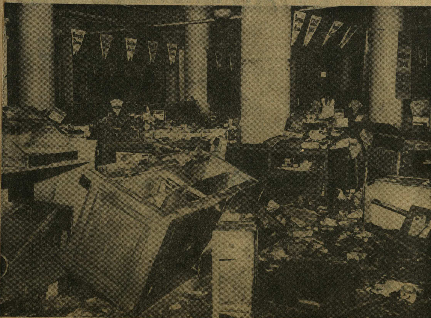
FLOOD AFTERMATH —Jumbled counters and merchandise-littered floors were left in Montgomery Ward's bargain department Wednesday as workers attempted
