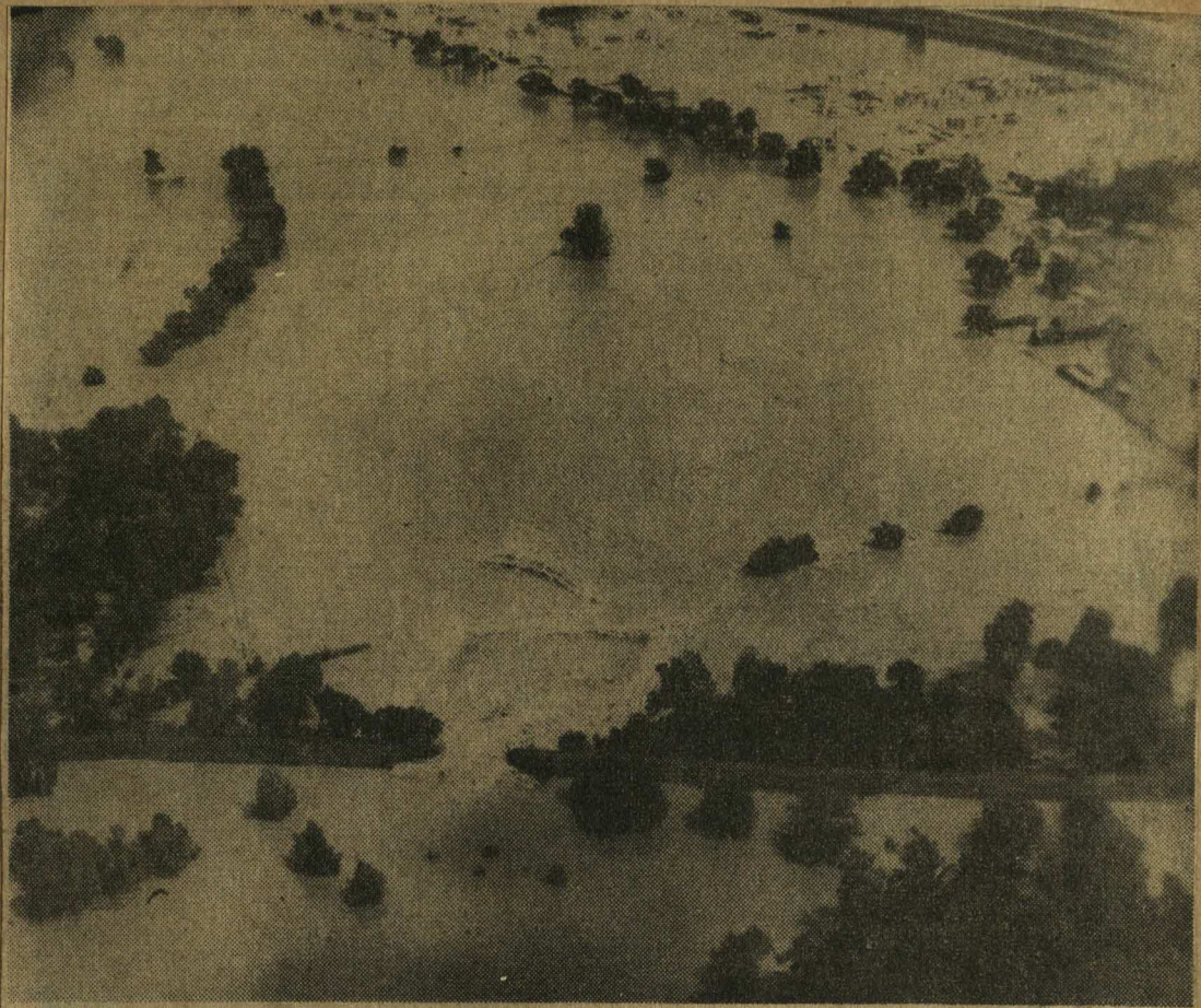
—Aerial Photo by Ed Ritchey. BREAK IN DAM —Boiling, muddy water spouting from this break (in center of photo) of Samuel Ave. levee flooded a number of homes on N. E. 10th, 11th, 12th, 14th and 15th Sts. Tuesday morning and forced evacuation of many Negro families. They waded to higher land, leaving possessions behind.
