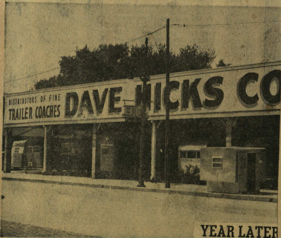
Apparently none the worse for the floodwaters, this business has been cleaned up. The owner, incidentally, did not ask or receive aid for his $100,000 damage.
