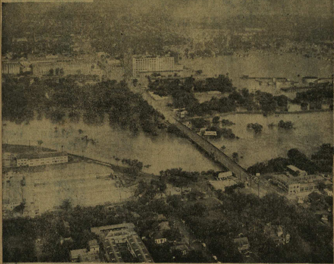
The Clear Fork spilled over a wide industrial area, flooding the Holly Plant of the city waterworks and all but isolating the western section of the city.
