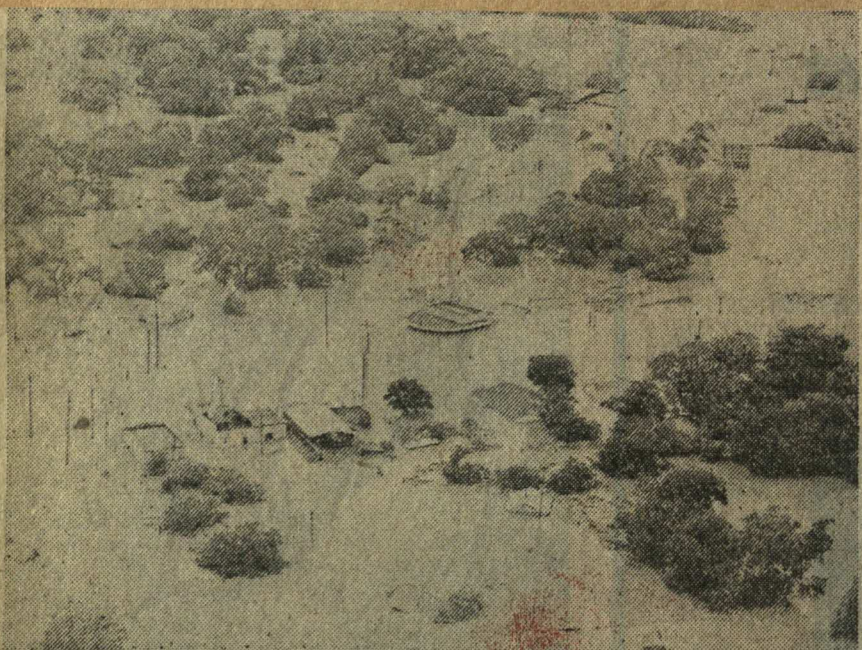
FLOODED . . . water covered businesses and homes at the intersection of White Settlement Road and Jacksboro Highway.
