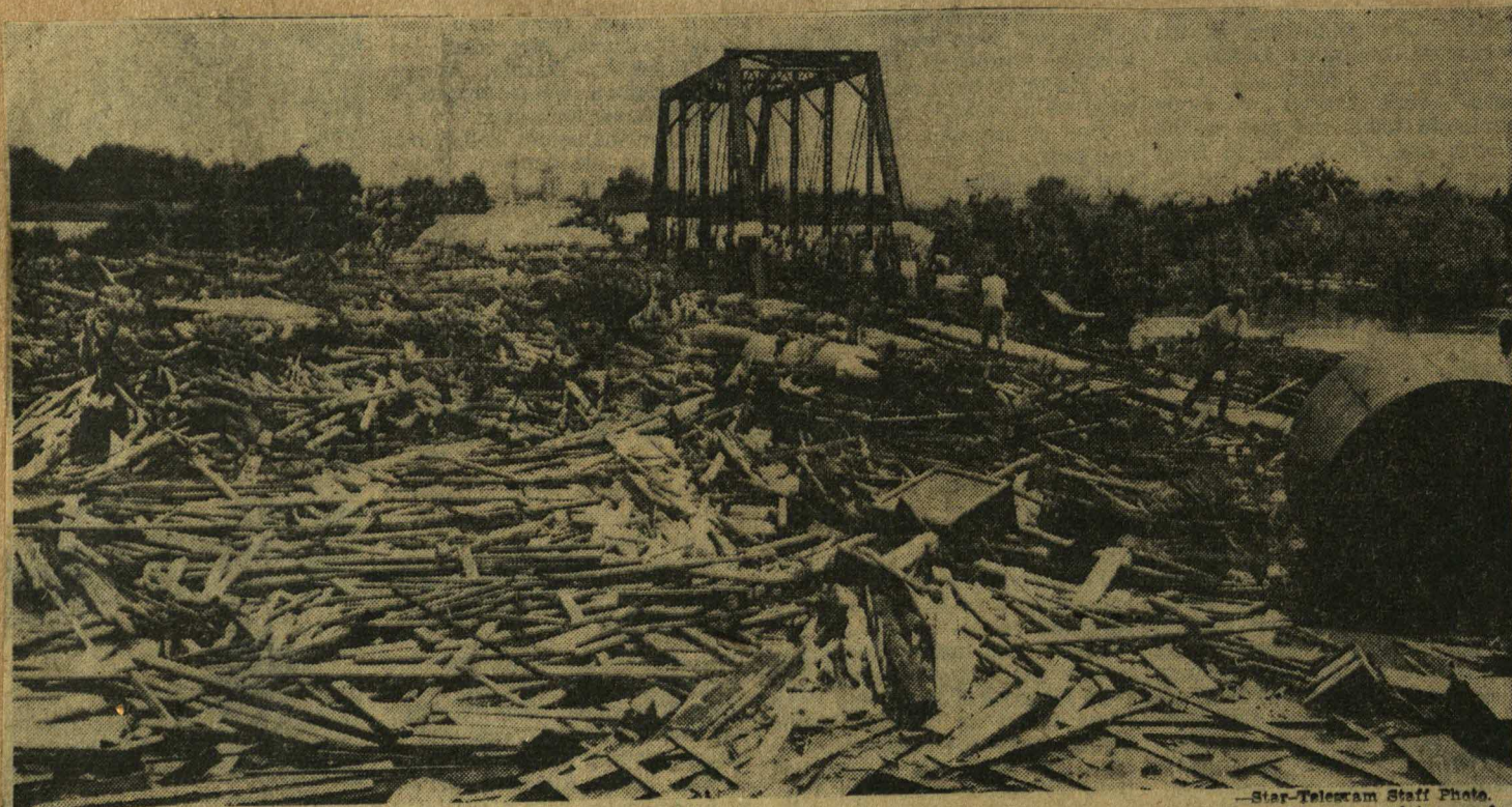
Debris is piled alongside the Frisco Railway tracks near the Texas Electric Service Company plant. Curious persons tramped over the area seeking anything of value. —Star-Telegram Staff Photo.
