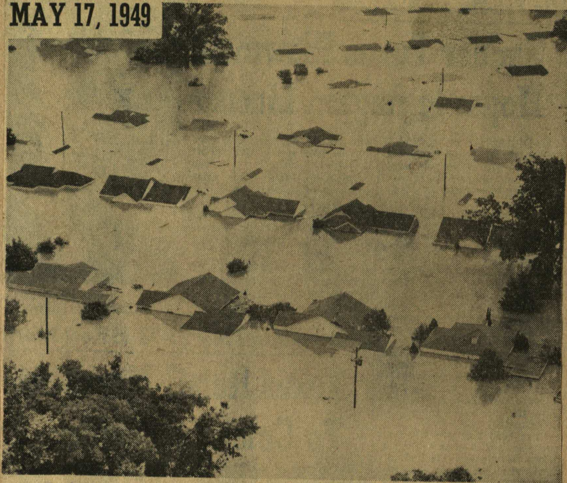
Rooftops here appeared like so many small islands in a sea. Residents took to the roofs for refuge until boats could take them to dry land.
