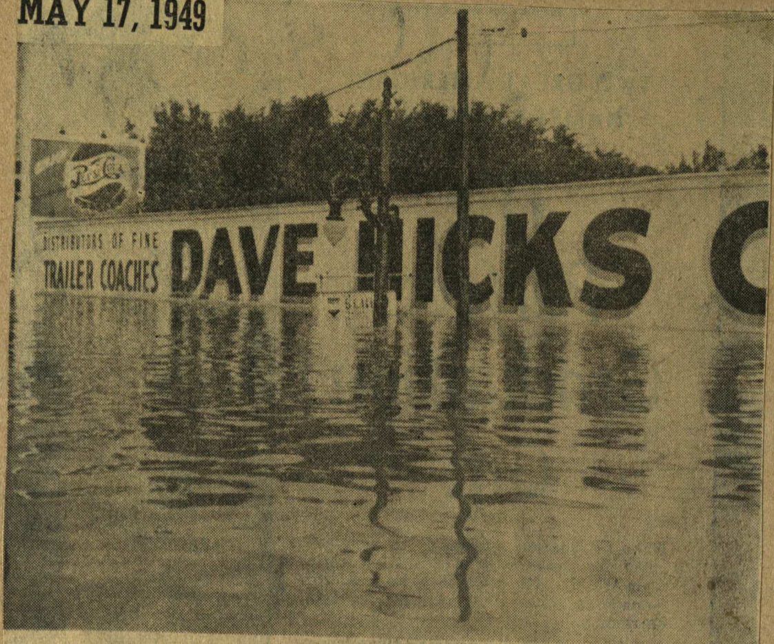
A very good idea of the depth the floodwaters reached can be had from this scene on West Seventh just west of the Van Zandt Viaduct. About 15 feet was measured here.
