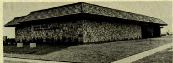
Constructed the Southwest Sub-Courthouse to serve residents of South and Southwest Fort Worth, and adjoining citizens.
