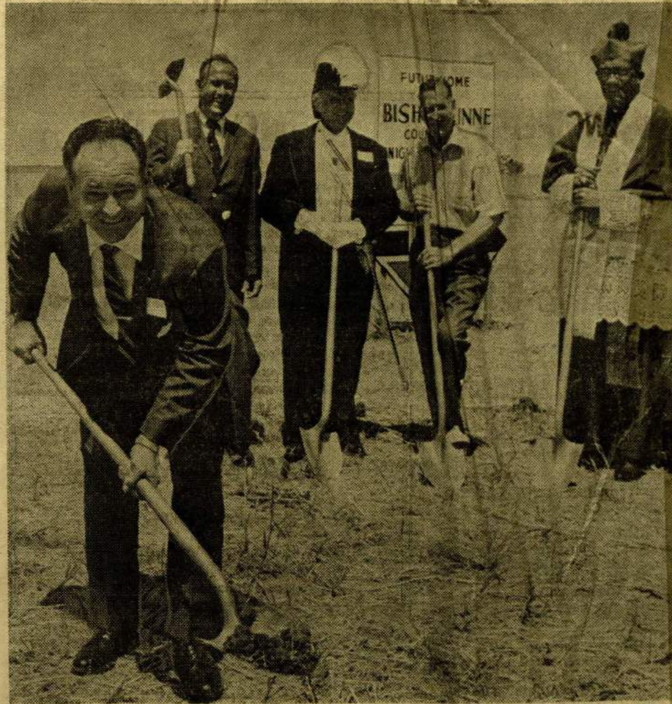
BREAKING GROUND—Eugene Urbano, Grand Knight of Bishop Dunne Knights of Columbus Chapter 2813, breaks ground Sunday for chapter's $90,000 Council Hall on Farm
