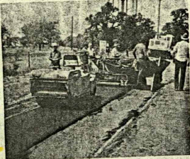
County workers put finishing touches on sidewalk.
