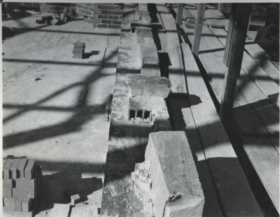
OCT. 14, 1949 WALL BOND STONE 9 M
