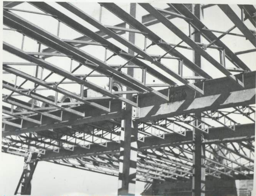
Nov. 1, 1949 - 2 ND FLOOR STEEL JOIST.
